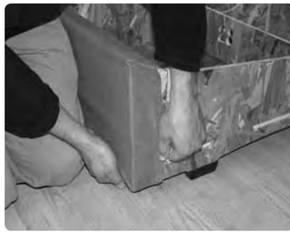
... and then pull the bottom corners of the cover around the bottom of the wood frame.
