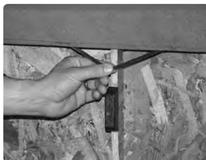
Reach up under the cover edge and pull out the little elastic bands...
