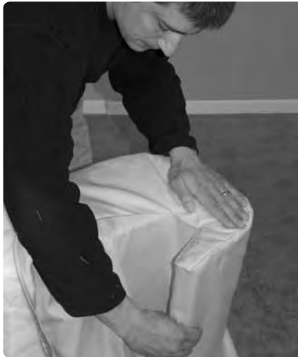
Fill in the wedge shaped area and the top of the cover. You can work the materials with your hands and also reach up under the cover to smooth and straighten.
