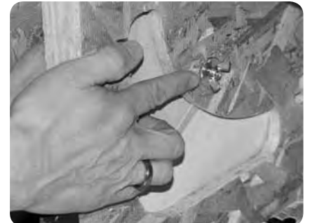
Take the washer and wingnut and get them started onto the bolt. Don't tighten completely.
