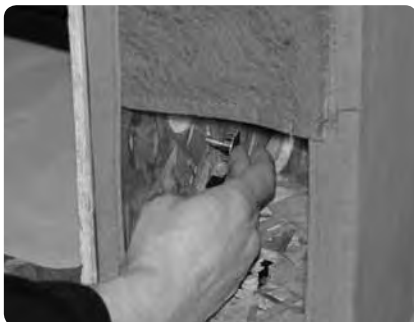
Reach inside the arm and insert the connector bolt into the hole.
