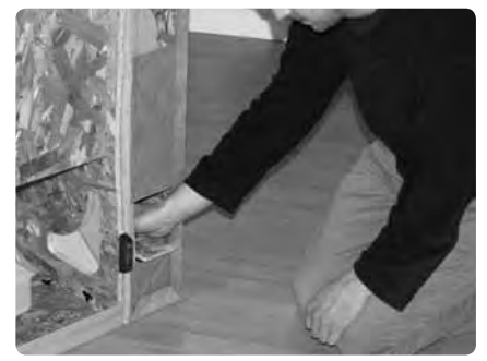
Follow the next steps to attach the connector bolt at the back of the frame (The hole closest to the floor with the frame on its back).
