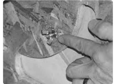
Take the washer and wingnut and get them started onto the bolt. Don't tighten completely.
