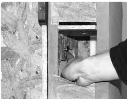
Now move to the top of the frame and put the next connector bolt in place.
