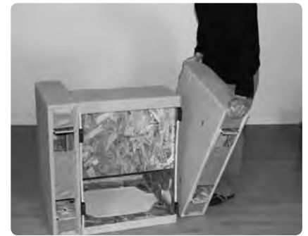
... and align them against the frame.
