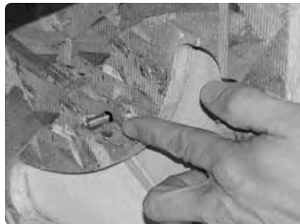
With the arm pushed against the frame, insert the connector bolt through the frame as shown.
