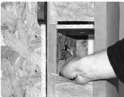
Now put the connector bolt that goes up at the front of the frame into place.
