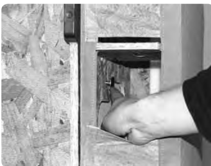
Now move to the top of the frame and put the next connector bolt in place.
