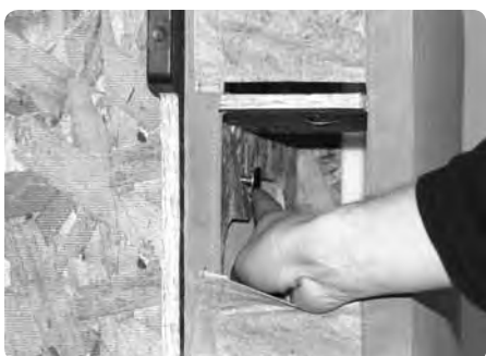
Now move to the top of the frame and put the next connector bolt in place.
